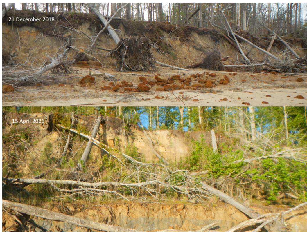
Fig. 9. Shoreline about 3 months and 34 months post-storm. Note ferricretes and storm terrace with only thin veneer of slope deposits (top), and thicker layer of slope deposits on eroded platform at bottom.
