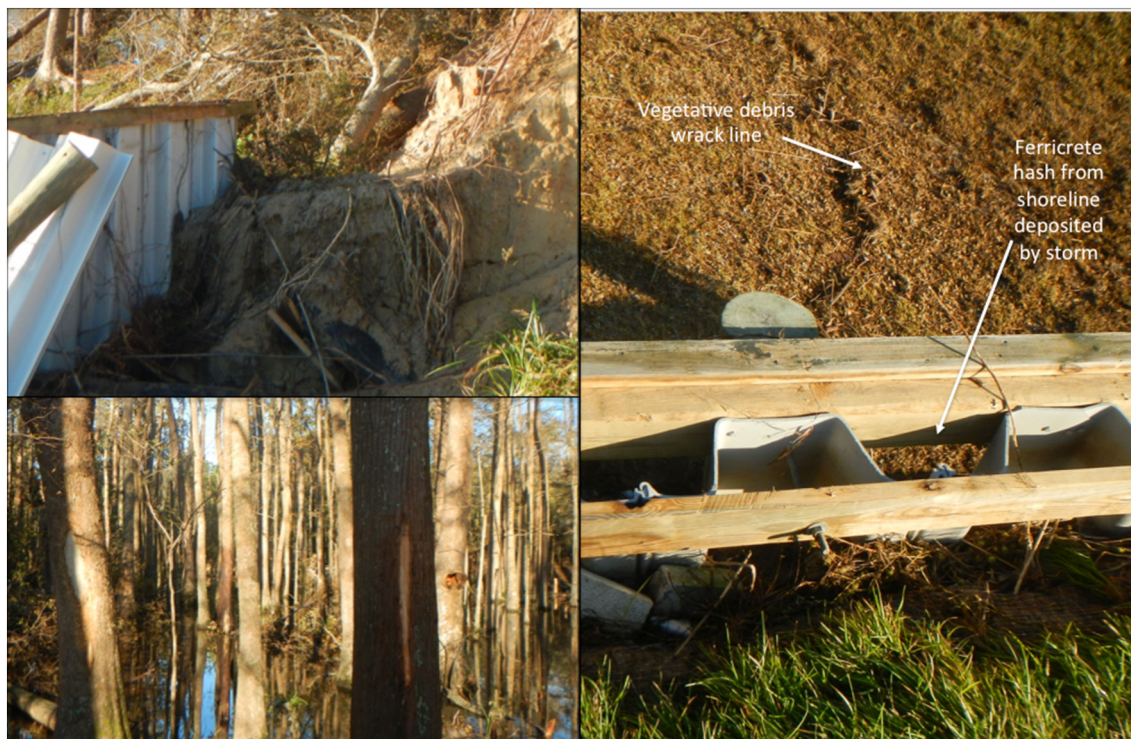
Fig. 5. Examples of storm high water indicators. Upper left: wave breaching of upper end of shoreline bulkhead tie-in. Lower left: Flood scars on swamp trees caused by abrasion from floating logs. Right: Shoreline bulkhead where cap board was removed by waves, with nearby wrack line and storm wave deposits.
